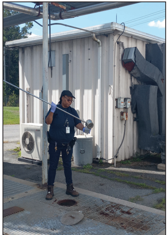
Marchelle Carter with Pine Bluff Arsenal's Directorate of Public Works checks water levels at the Arsenal's Central Waste Treatment Plant.
