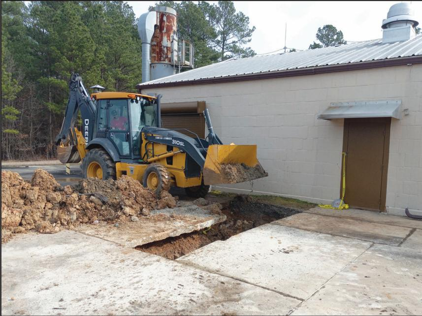
Scotty Bridges, with Pine Bluff Arsenal's Directorate of Public Works Pipe Shop, repairs pipe and replaces a broken water main valve at an Arsenal building.
