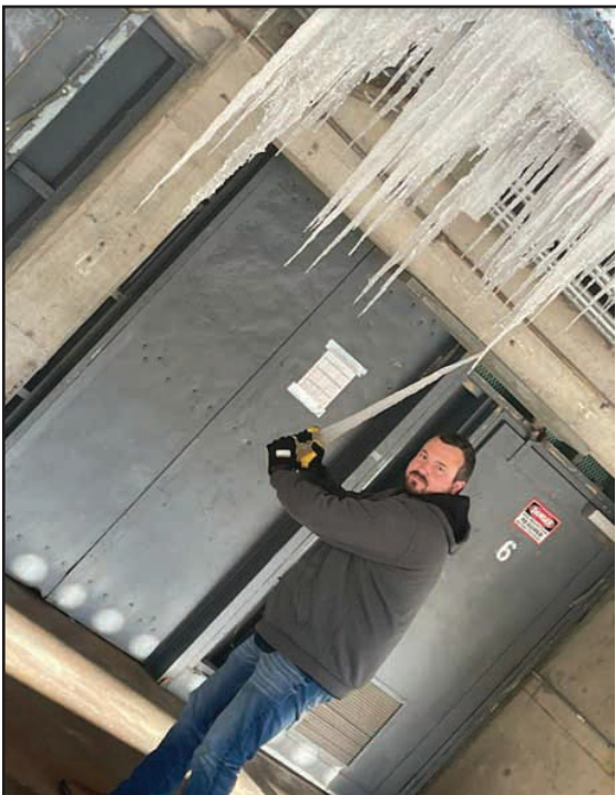
Brad Dobbins, Utilities Operator Leader, with Pine Bluff Arsenal's Directorate of Public Works, has a little fun with an icicle from the edge of a production area roof, while valving off a water leak due to the recent winter storm. U.S. ARMY PHOTO-DPW
