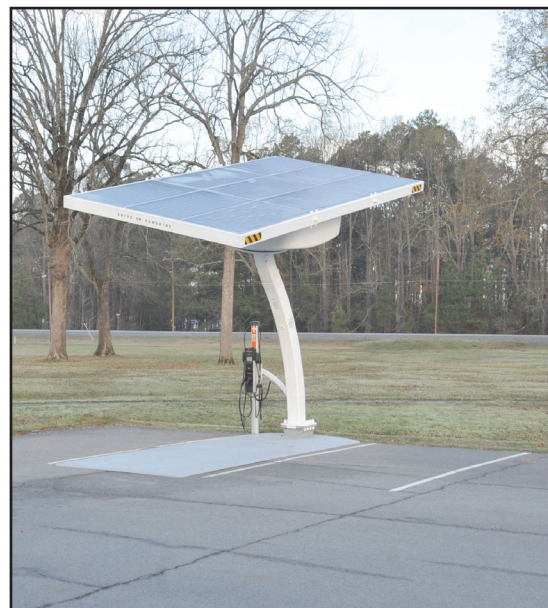
One of five solar electric car charging stations on Pine Bluff Arsenal. U.S. ARMY PHOTO BY HUGH MORGAN
