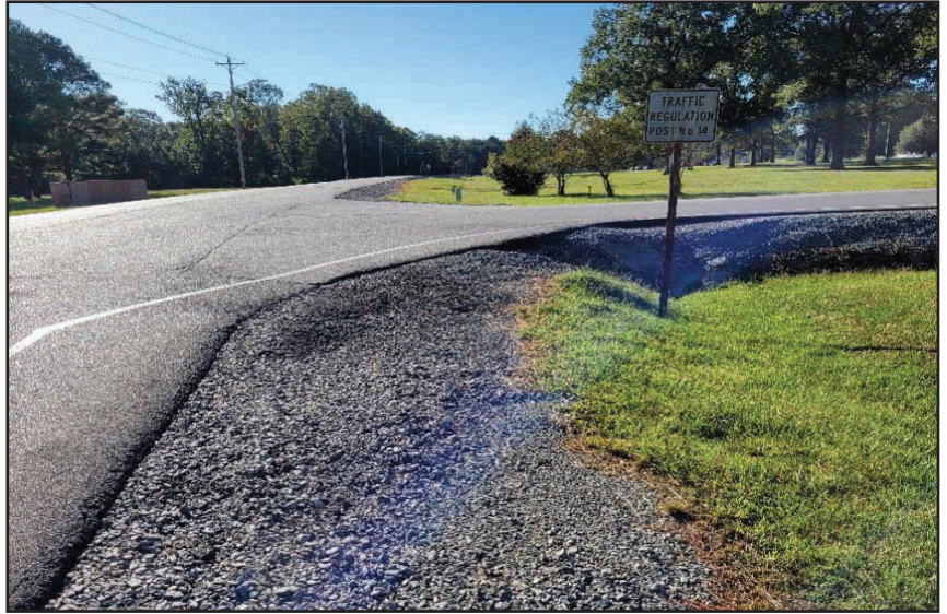
Photo above, SOP information shows Sibert/Wise Road intersection needs widening on the shoulder so there can be proper run off and drainage.
