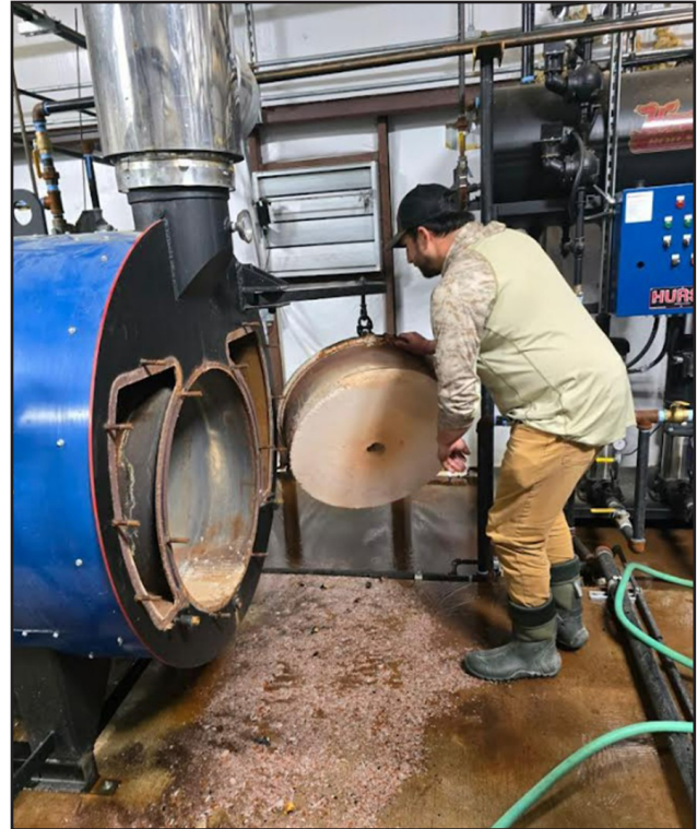
Cory Dejarnette, photo left and Tyler Cox , photo right, both Boiler Operators with Pine Bluff Arsenal's Directorate of Public Works open up boilers for an annual boiler inspection. U.S. ARMY PHOTOS BY DPW
