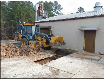
Scotty Bridges, with Pine Bluff Arsenal's Directorate of Public Works Pipe Shop, repairs pipe and replaces a broken water main valve at an Arsenal building.
